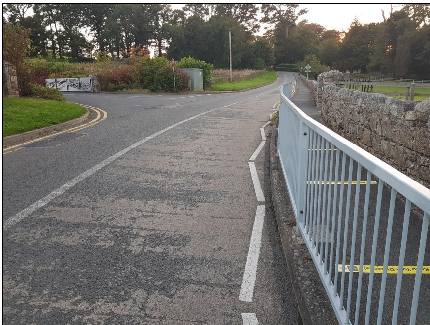
Figure 4.1: Existing Footpath on Cookstown Road
