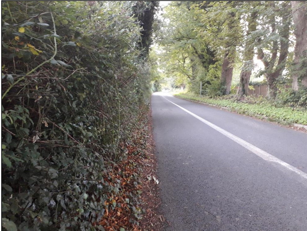
Figure 4.1: Steep roadside cuttings and dense vegetation on Cookstown Road, which may restrict a cyclist from keeping clear of motorists if needed
