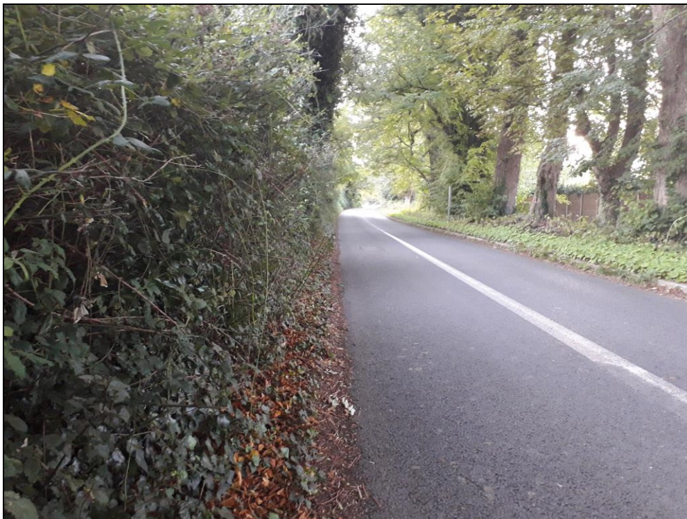
Figure 4.7: Steep roadside cuttings and dense vegetation on Cookstown Road, which may restrict a cyclist from keeping clear of motorists if needed
