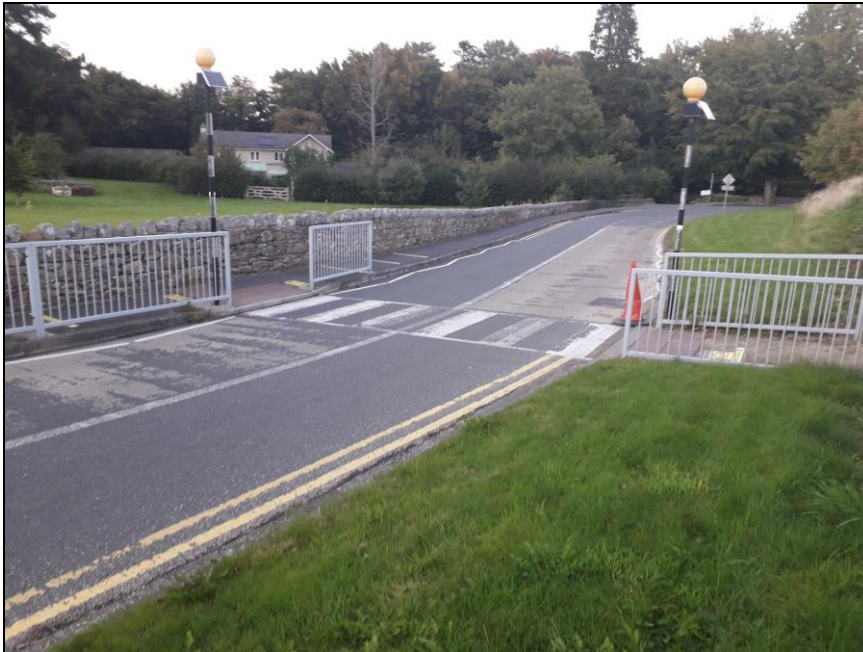
Figure 4.2: Worn and missing road markings at existing Zebra Crossing on Cookstown Road
