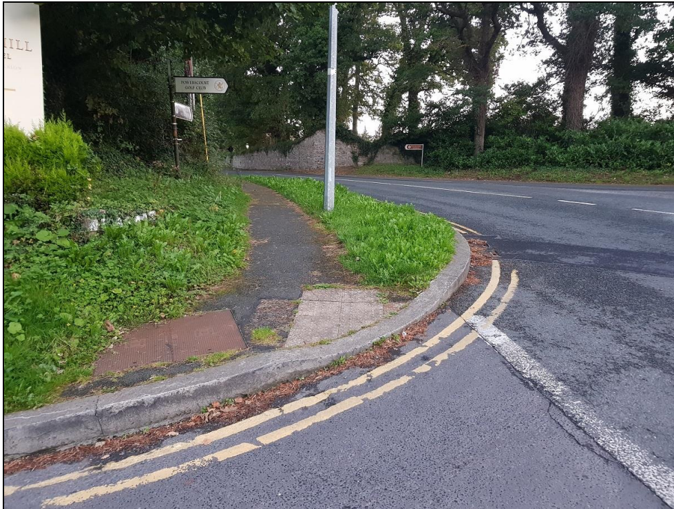
Figure 4.6: Visibility to left limited for road users, including cyclists, at R760 / Cookstown Road junction
